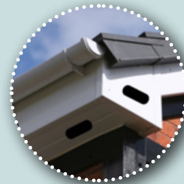
Potential locations for nest entrances in a standard fascia and soffit.
